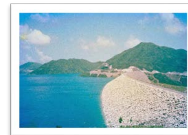
Areas around the west dam of the High Island Reservoir in Sai Kung (the late 1970s) (Reference no.: HKRS572-2-3)
